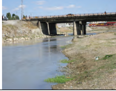
Photo 2 - Station 1 The Murat River bridge.
