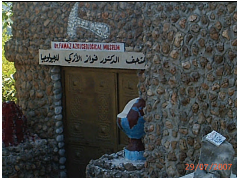
Figure 5. Entrance to the Museum Building (original).
