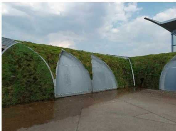
Figure 3. Bioactive facades for rainwater management implemented at the Therme wellness complex (original).
